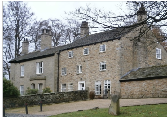
P5.2 Pott Hall, the right hand side is three storey
