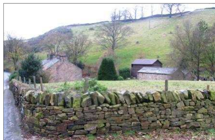
P3.3 Group of buildings at Pott Mill (outside the National Park)
