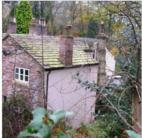
P6.10 Stone slate roof and brick chimneys at Harrop Close, the brick gable, rendered rear
