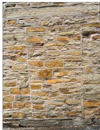
P5.7 Evidence of a blocked doorway
