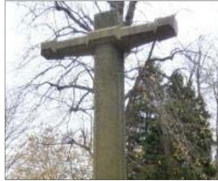
P5.6 The Cross transom is a later addition
