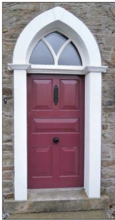
P5.12 Nineteenth century style door at Pott Hall Farm
