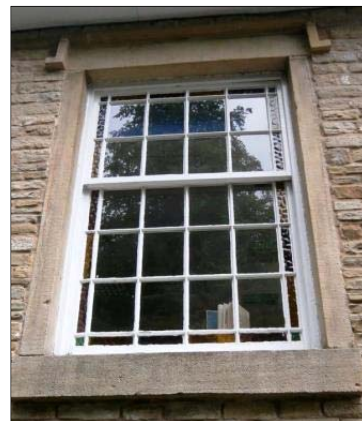
P5.10 Nineteenth century sash window with hoodmould at the school
