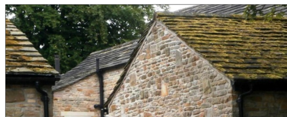
P6.6 Stone slate roofs at Pott Hall
