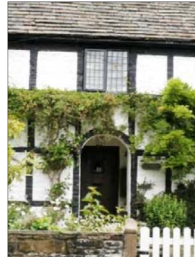
P6.3 The Croft is painted to resemble a timber frame building.
