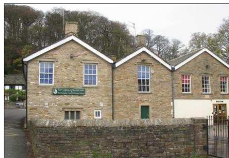
P3.9 Pott Shrigley Primary School, the original building is on the left
