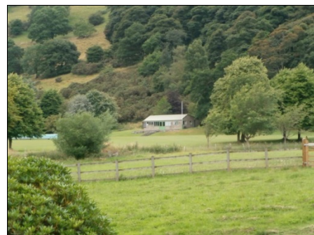
P5.20 The rebuilt Cricket Pavilion
