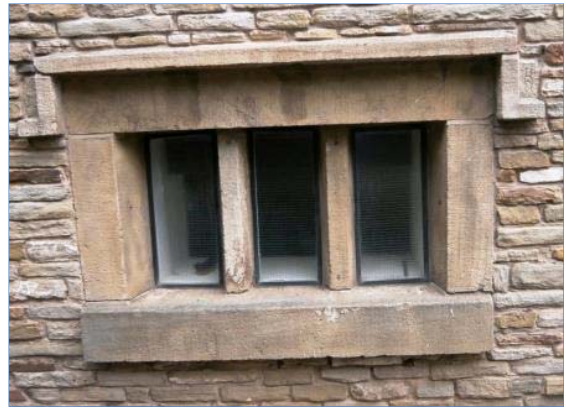
P5.9 Nineteenth century mullion window with hoodmould over
