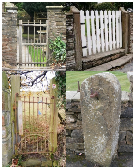
P6.17-20 A variety of styles of gates and piers can be found in the Conservation Area
