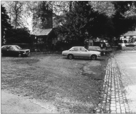
P1.1 The car park before re-surfacing (above)
